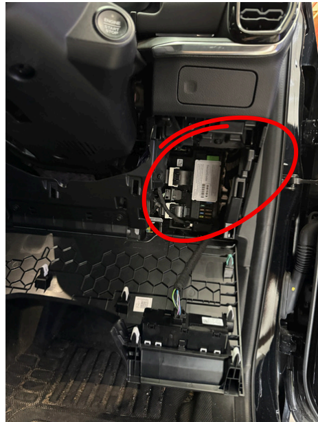
Fuse box Location
